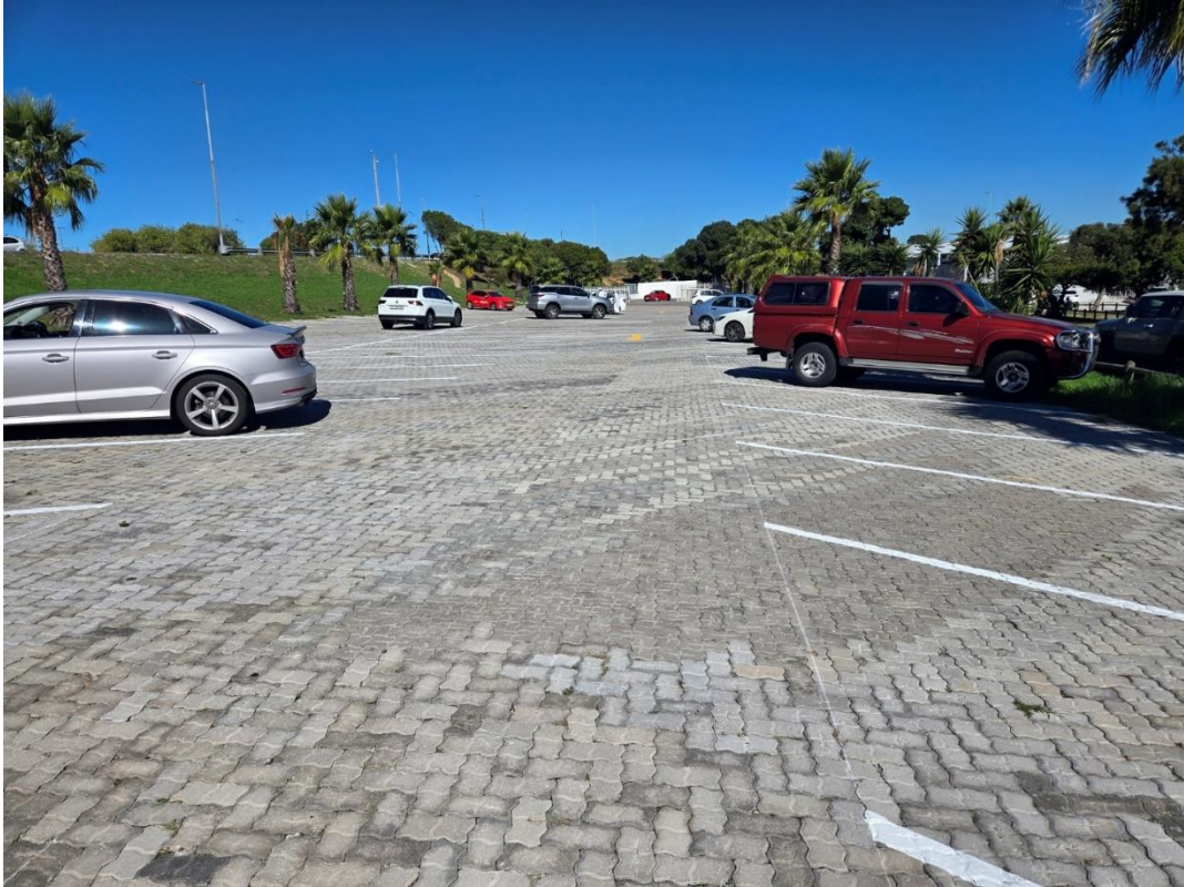
Figure 2 – External Parking area paved with parking bays painted.
