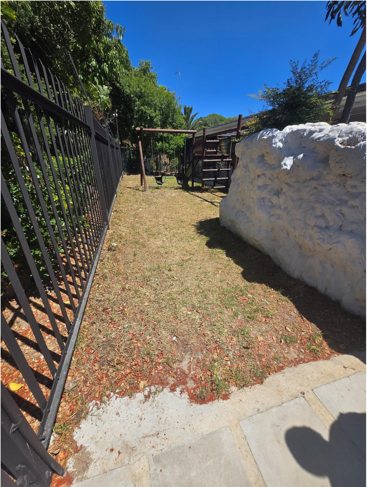
Fig 6. Play Gym successfully relocated (View before Astro-Turf was installed.)
